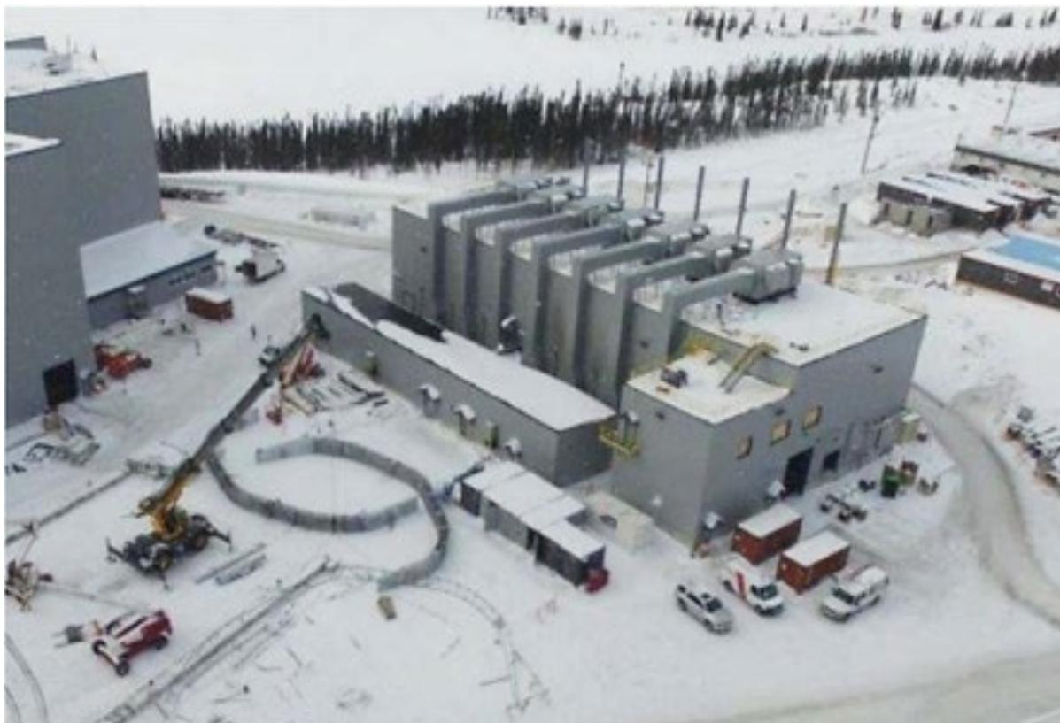
*Image 4. LNG-fired power station with a total capacity of circa 16MW.*
