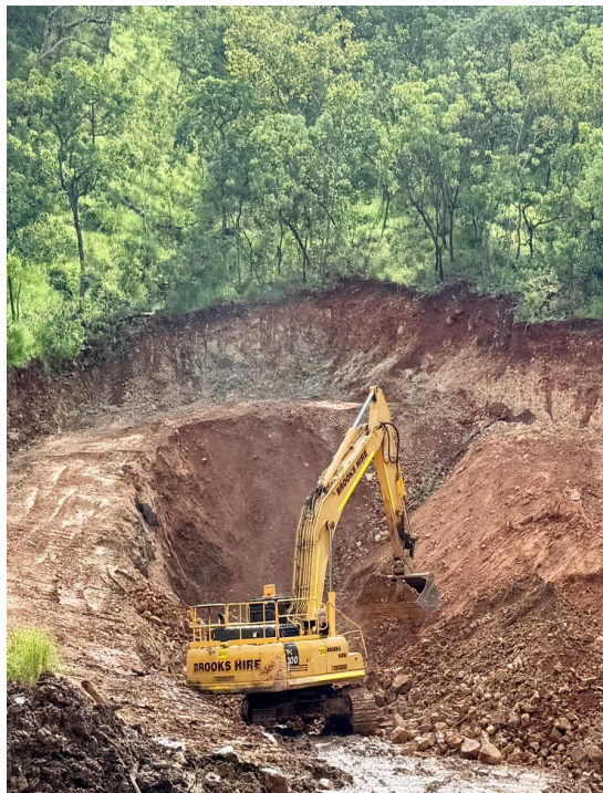
Plate 1 – Ground stability and box cut earth works
