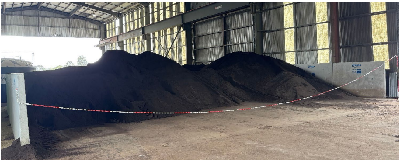
Ash received and stored in Ash Bunker ready for start-up
