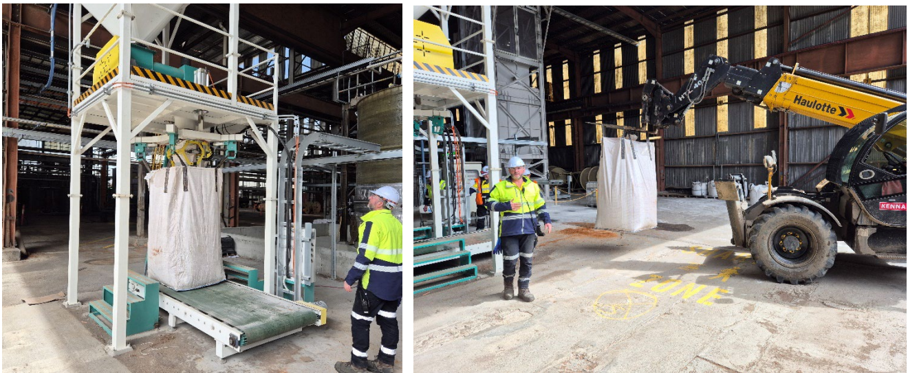
Loading of MgO into 1t bags (left) and relocating bags to storage area (right)
