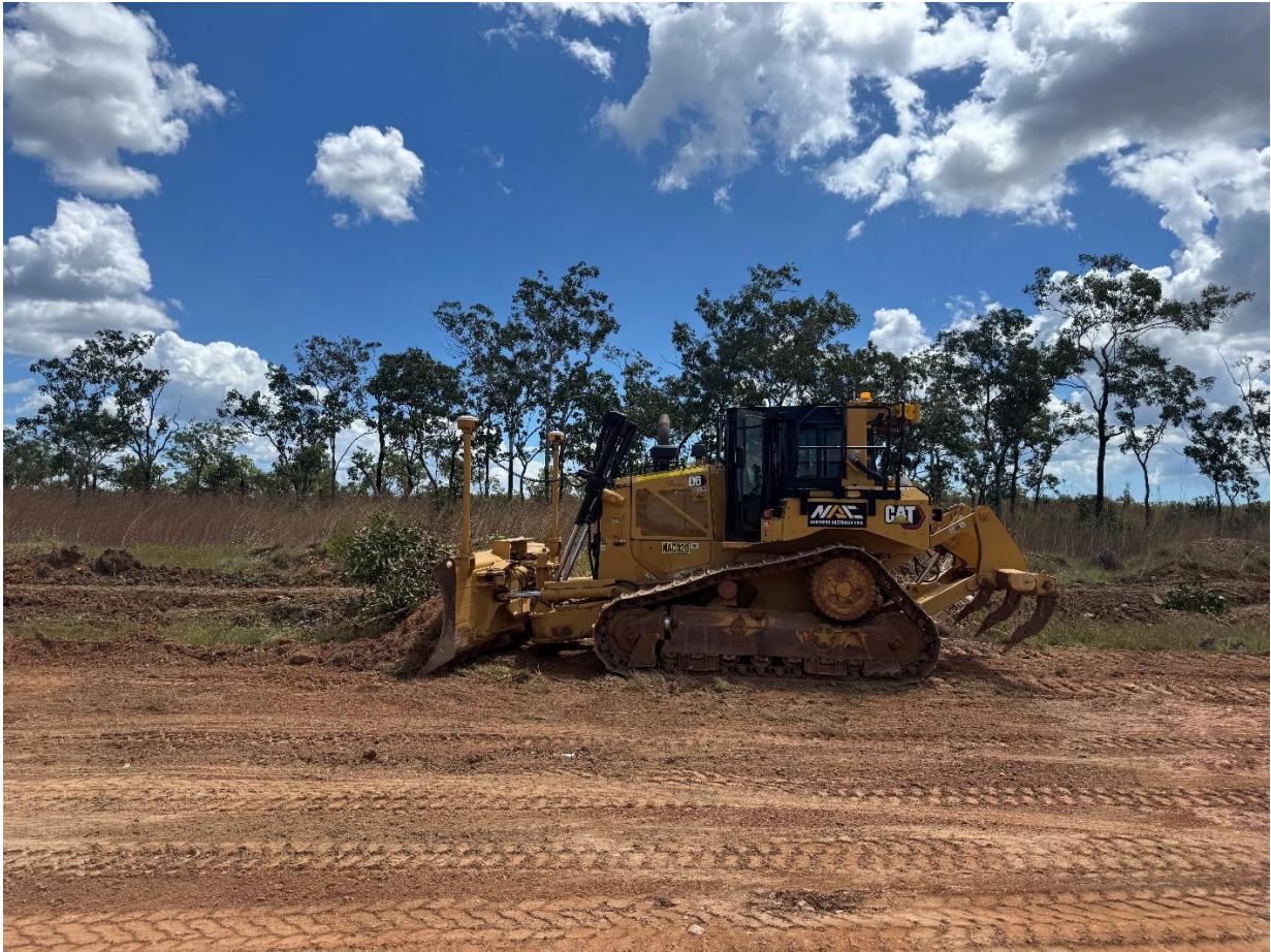
Figure 1 BP33 early works underway
