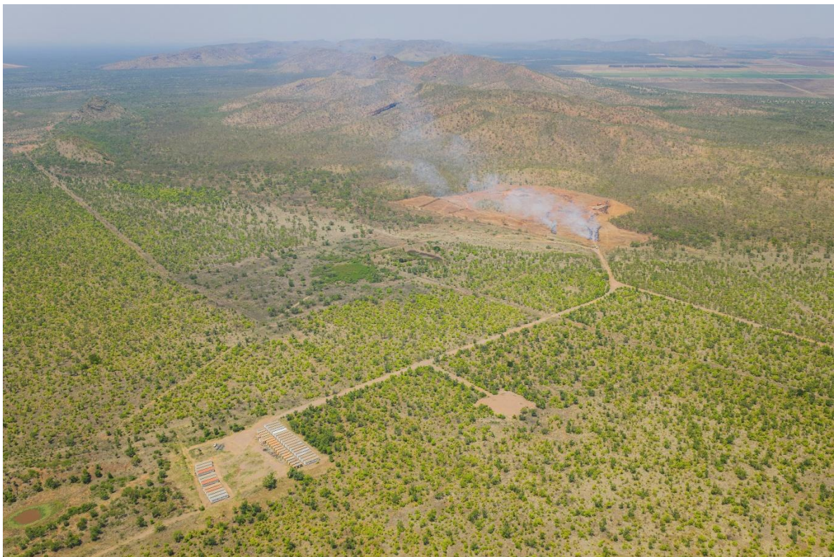
Figure: Clearing for Processing Plant with camp infrastructure in the foreground
