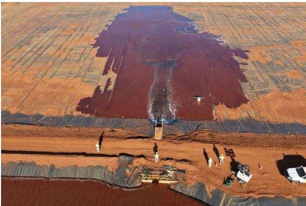
Figure 2: Filling of the first crystalliser
