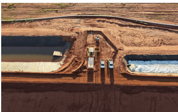
Figure 5: Lift station two commissioning
